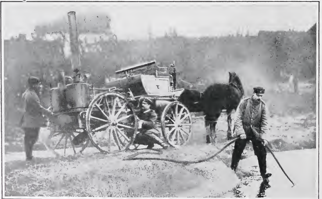
WITH THE GERMAN ARMY. Portable filter and sterilizer.
