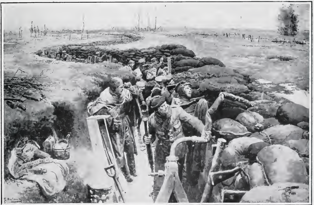
IN THE FLOODED TRENCHES.
