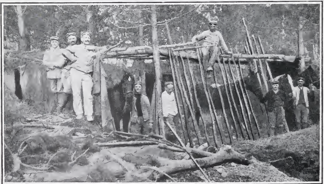
GERMANS ERECTING SHELTERS.
