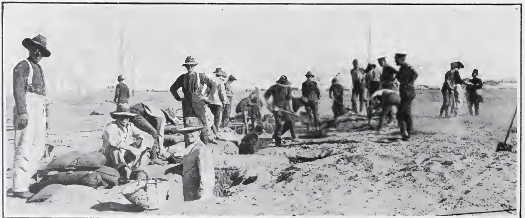
A PARTY OF THE NEW ZEALAND CONTINGENT Trench-digging in the desert.
