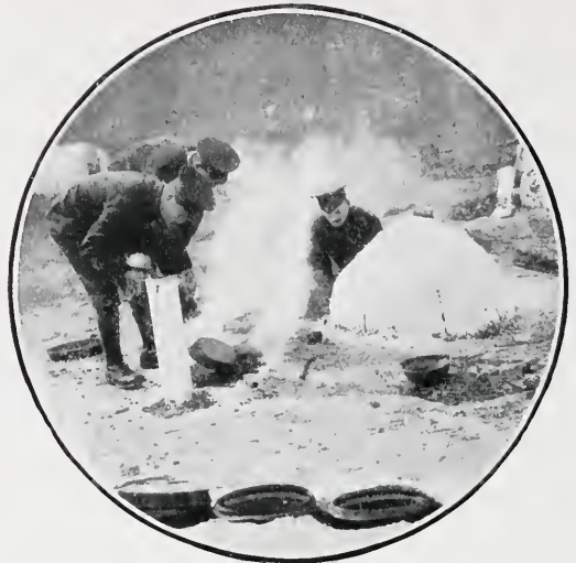
PLACING A JOINT INSIDE A BEEHIVE OVEN.
