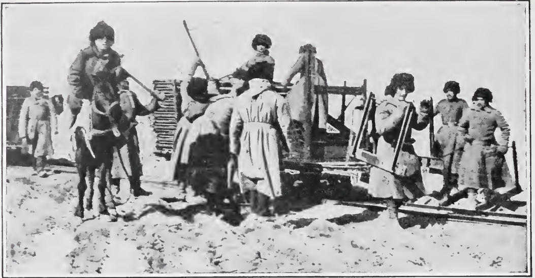
RUSSIAN ENGINEERS AT WORK. Constructing a railway track for transports.
