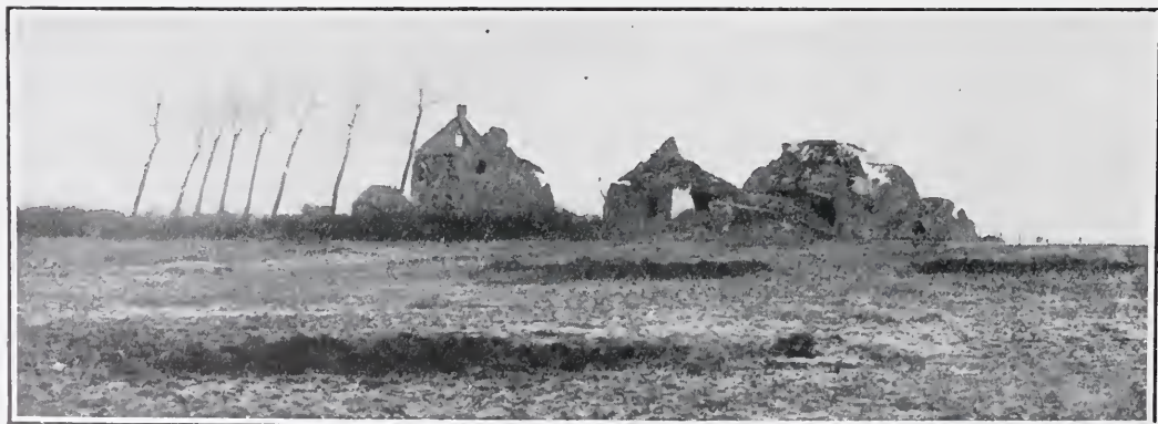
RUINED BUILDINGS AT ST. ELOI.
